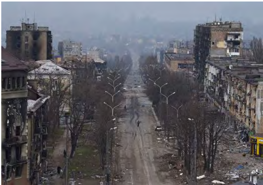
A view shows buildings damaged in the southern port city of Mariupol, Ukraine, April 3. REUTERS/Stringer
