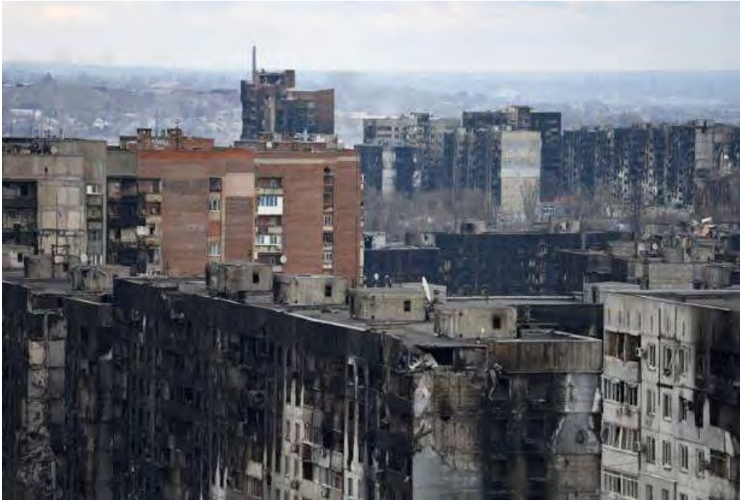
A view shows apartment buildings damaged in the southern port city of Mariupol, Ukraine April 4. REUTERS/Stringer
